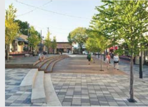
Paver Plaza with Concrete Banding
