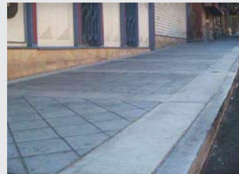
Pavers with Concrete Banding
